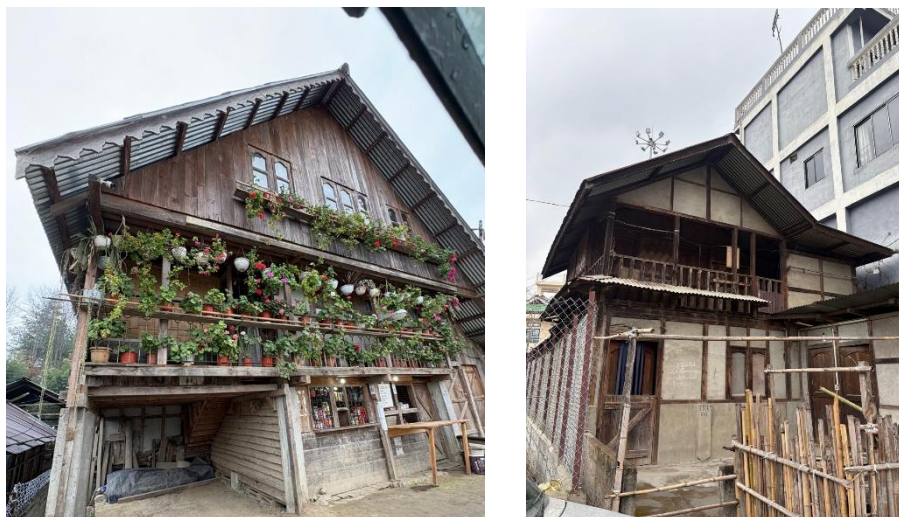
Fig. 18: Traditional Apatani House and Modern RCC Building
