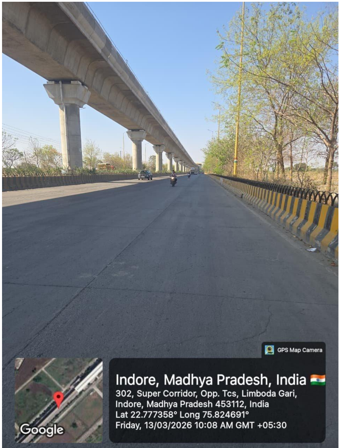
Fig. No. 7 field survey metro photos
