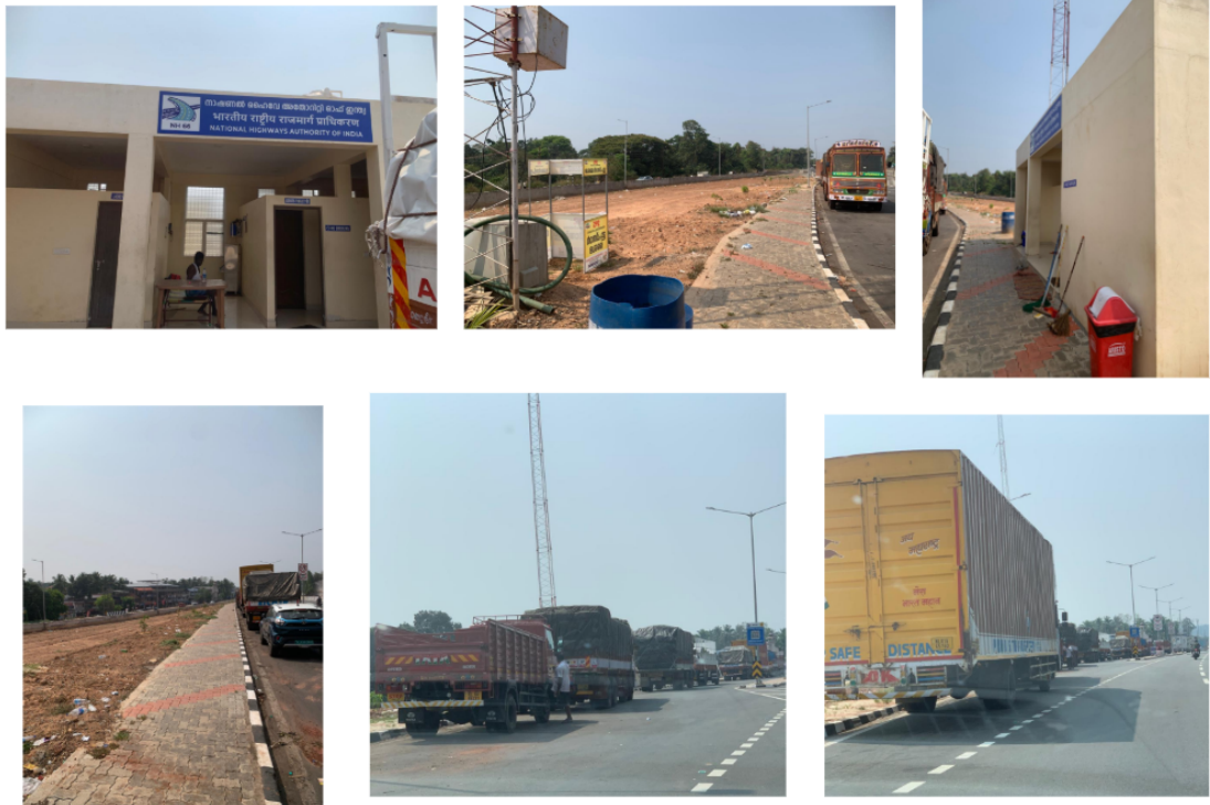
Fig.1.3 Site condition on NH-66,Kohinoor, Malappuram
