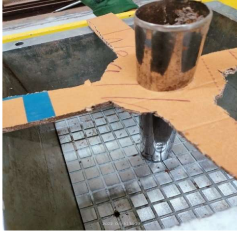
(a) Placement of steel Pipe at the center
