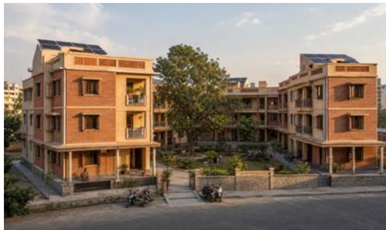
Fig. No. 6.1: Zone A: Rehabilitation housing design concept. U-shape cluster layout with open central courtyard, raised plinth, cross-ventilation, and front verandas. (AI-generated design intent illustration for conceptual reference only)
