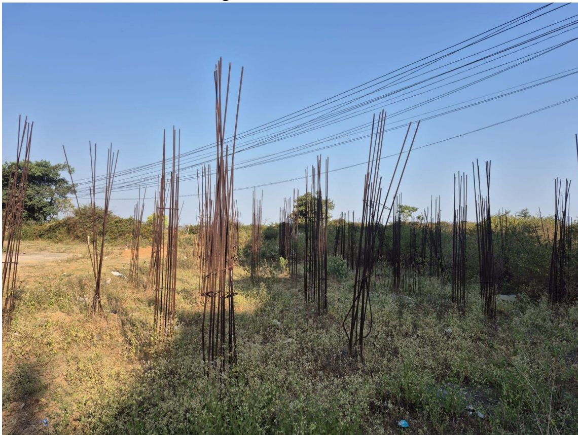
Image 2. Under constructed site
