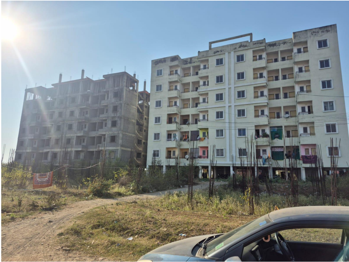
Image 1. Under constructed sites
